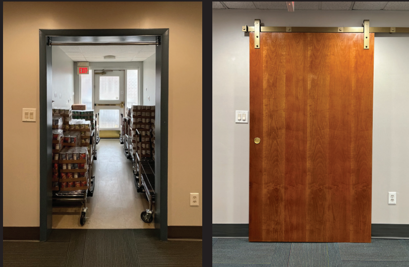
Barn Door Installation Project 2025
